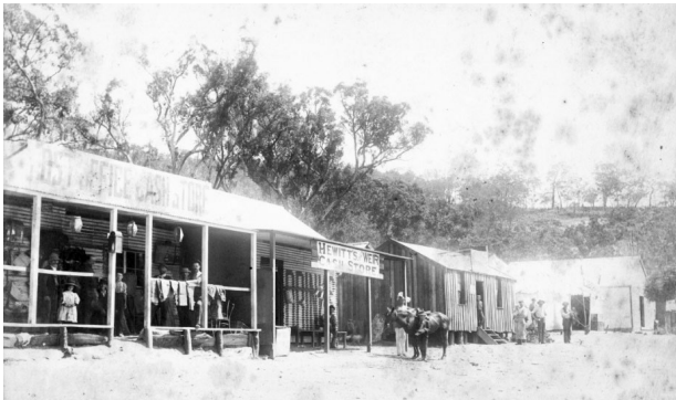
FIGURE 4: HUMPHREYS STORE, MUNDARING WEIR CONSTRUCTION CAMP C. 1900. Courtesy: SLWA b2267271_1.
