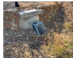
Slotted basin outlet structure to slow stormflows
