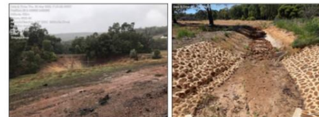
Extended detention basin Gidgegannup
