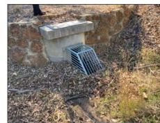
Slotted basin outlet structure to slow stormflows
