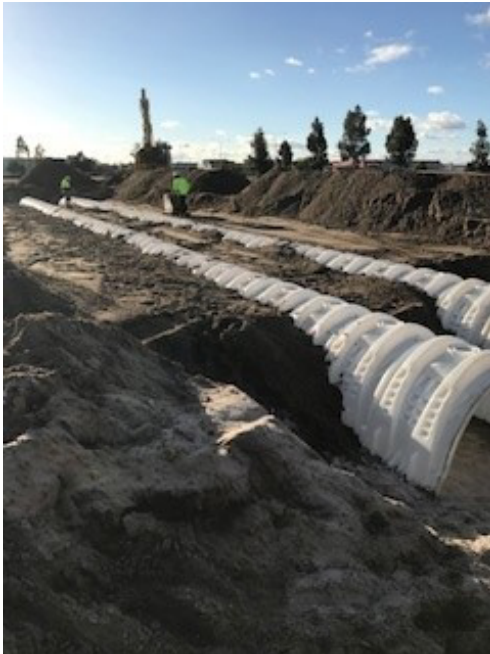
Picture showing backfilling.
