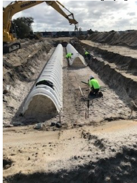
Picture showing laying.
