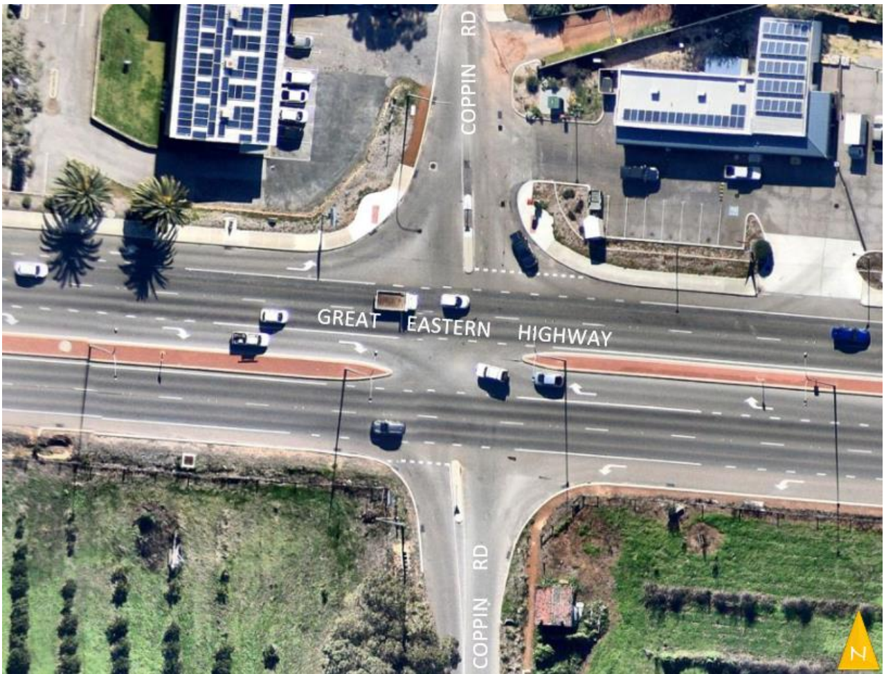
Photograph 1 – Coppin Rd/ Great Eastern Hwy intersection (KI1) Aerial
