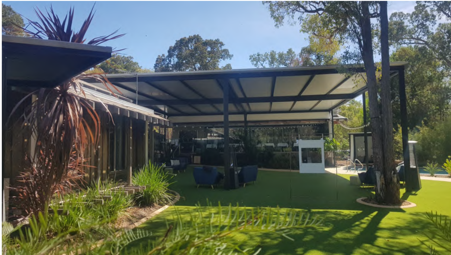
Figure 7: Photo of the restaurant building and patio.
