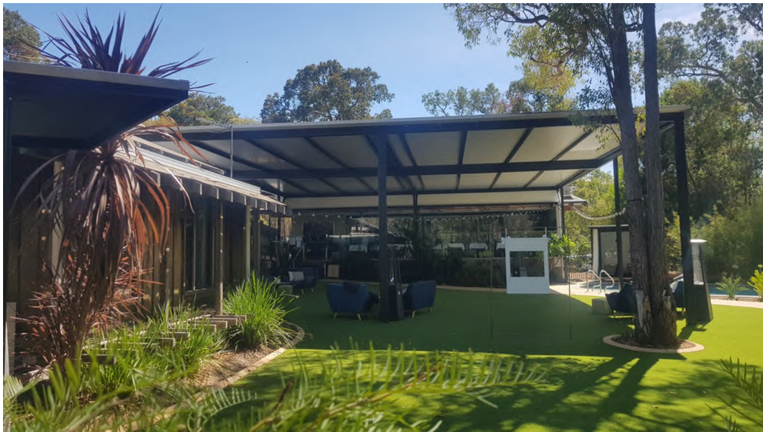
Figure 7: Photo of the restaurant building and patio.
