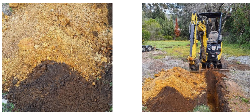
Figure 4.9 (L) Spoil. (R) Excavation of TP2.
