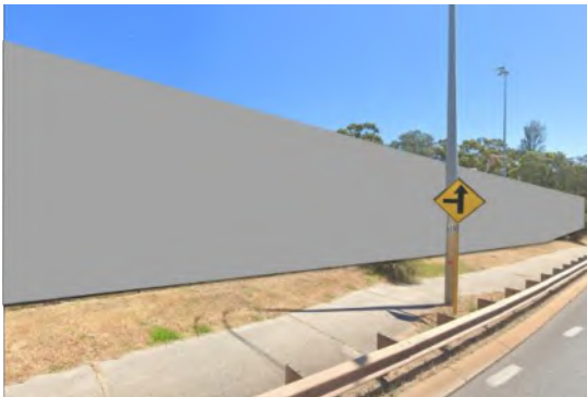
View of Bilgoman Aquatic Centre with concrete sound wall twice the height of current fence.
