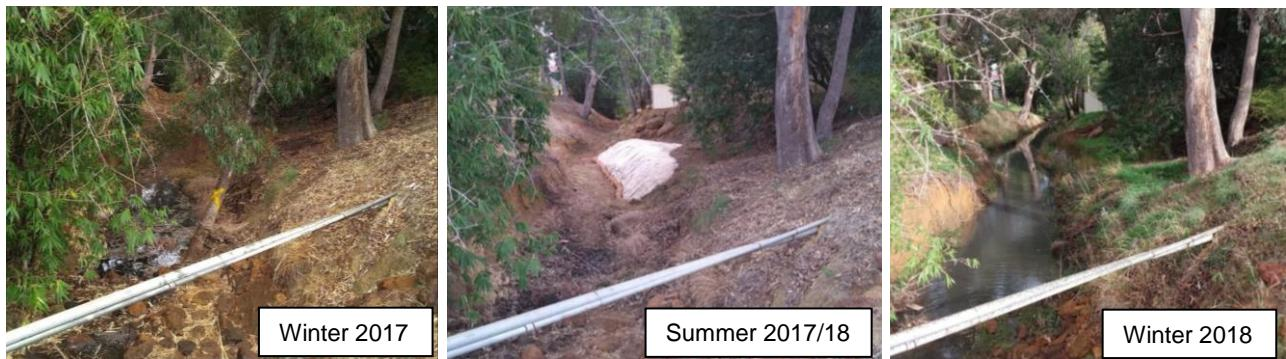
The above images were taken at 6 month intervals before, during and after installing a riffle in a watercourse to slow water flow, as part of a restoration project. The pipe in the foreground provides a clear reference point for comparison, as does the tree on the right.
